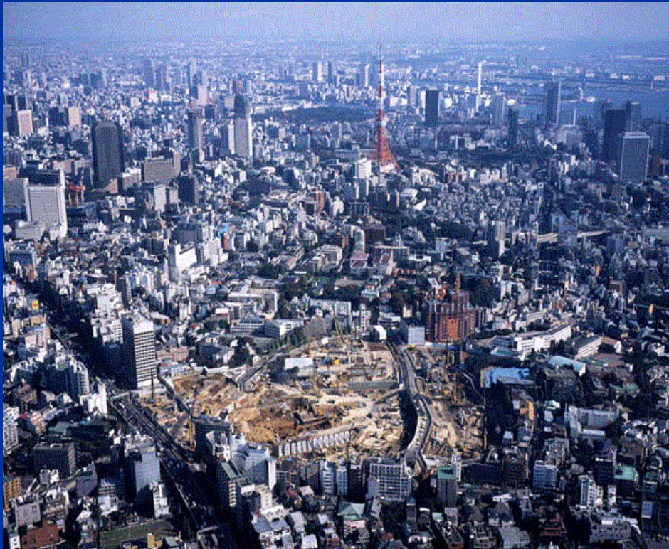
Project Site in Tokyo (2000)
